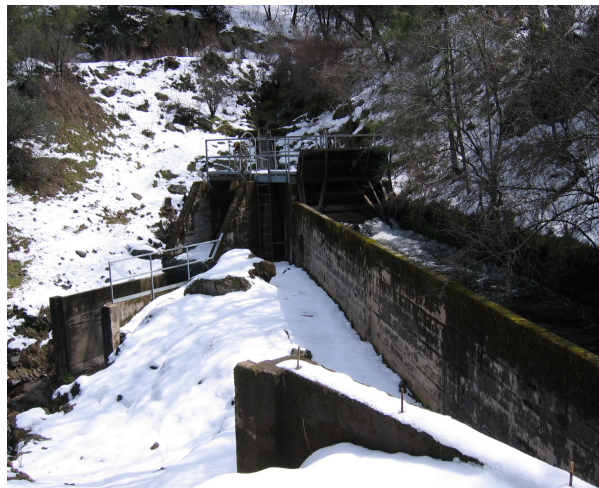
Stanislaus Forebay tunnel & secondary spill channel
