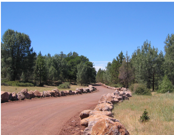
Road at Pit 1 Forebay
