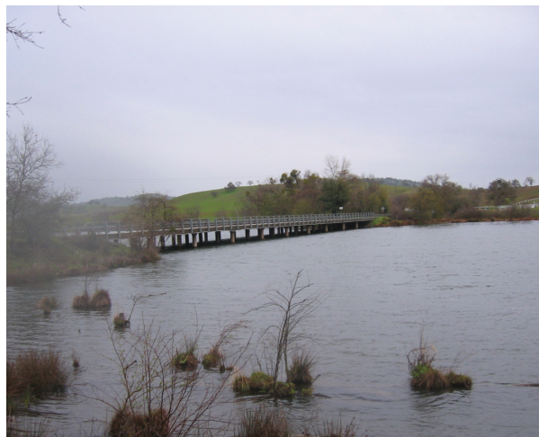
County bridge over the Merced Falls Reservoir
